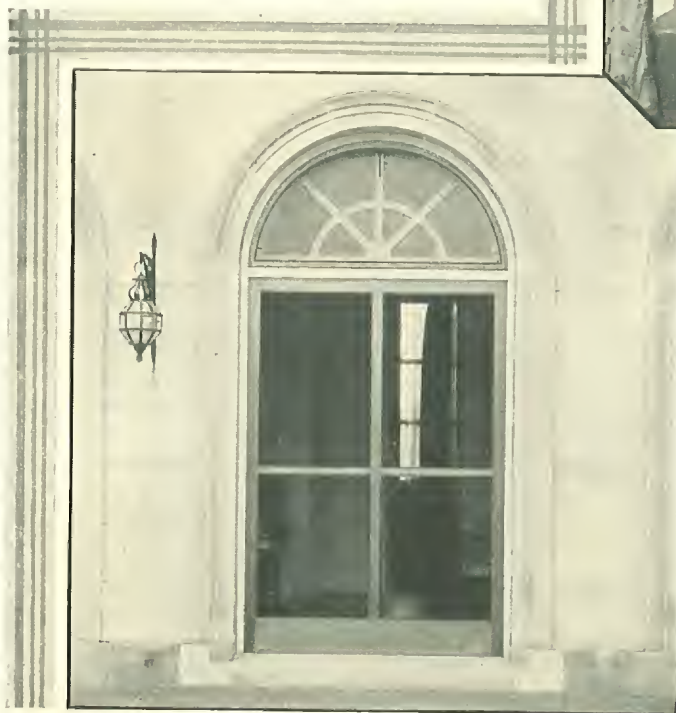
(Left)—Fixed panel outside where full length casement opens in. Transom also is screened. Panel is readily removable.
